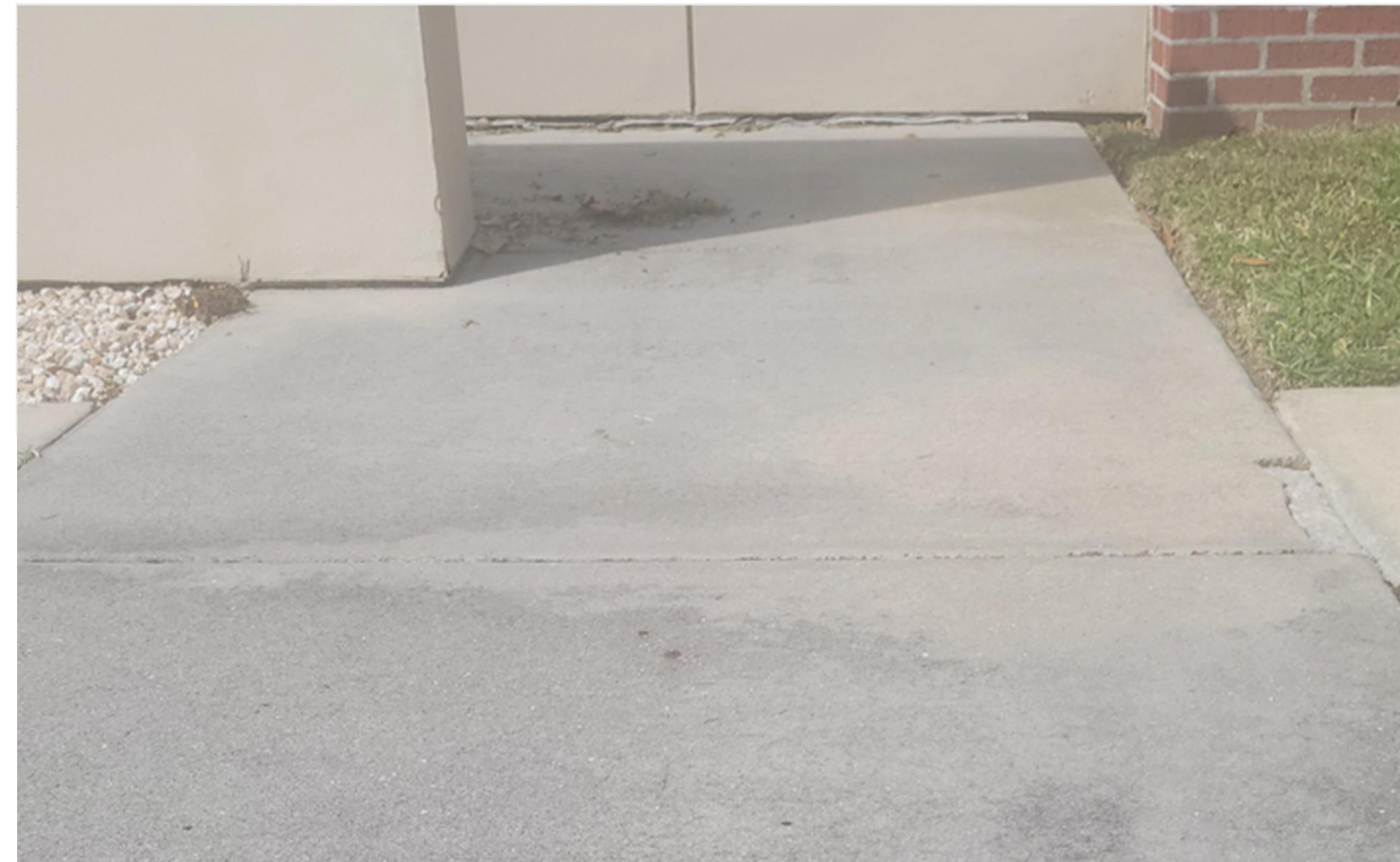
BOTTOM SLAB, LOOKING WEST. NO VISIBLE DISPLACEMENTS AT ADJOINING SIDEWALKS.
